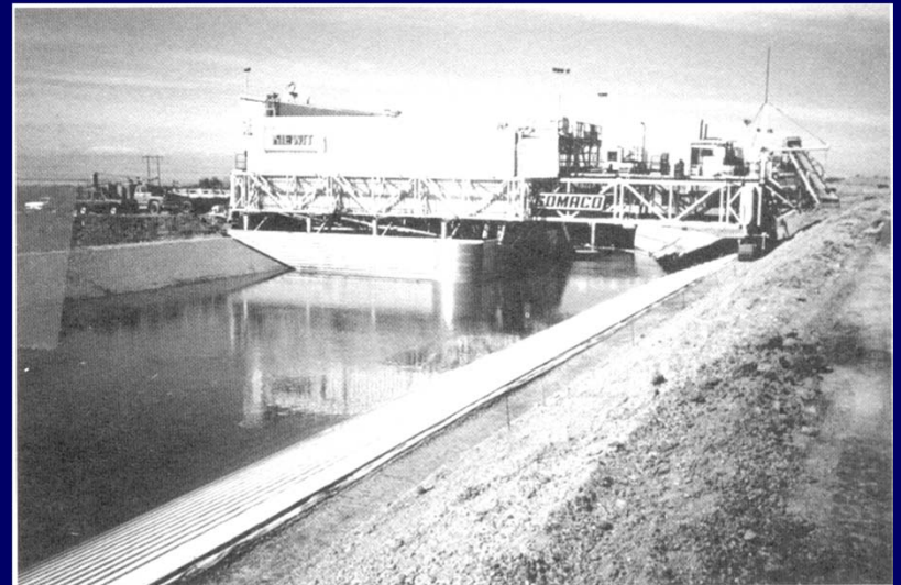
(Lining a "Live" Canal)
