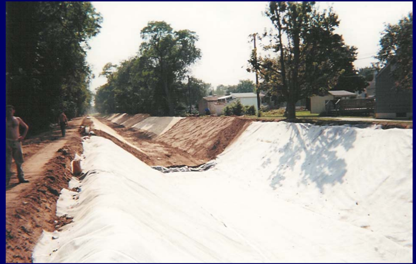
(GCL Lining of a Canal)
