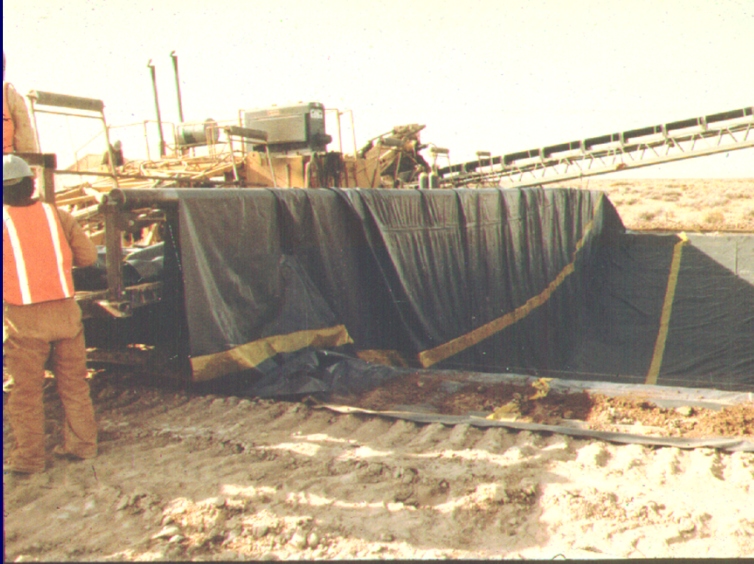
(Lining a Canal: Before Soil Covering)
