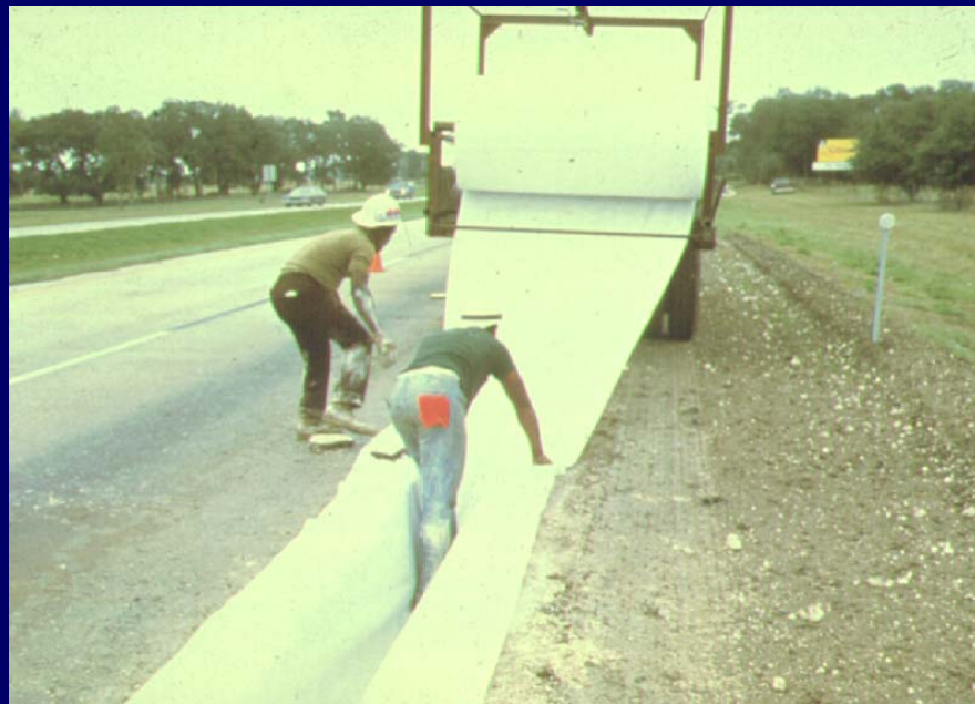
(GT Filter in Excavated Trench)
