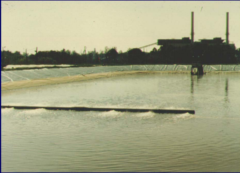
(Double Lined Hazardous Waste Pond)
