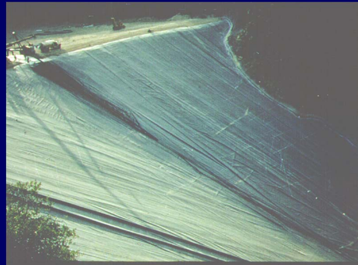
(Lined Earth Dam: Before Rip-Rap)
