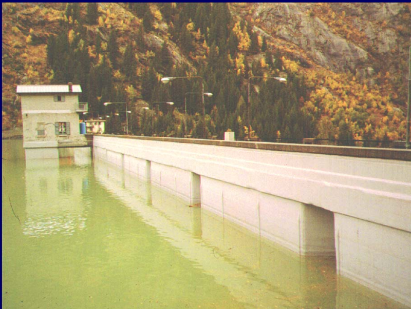
(Completed Concrete Dam Lining)
