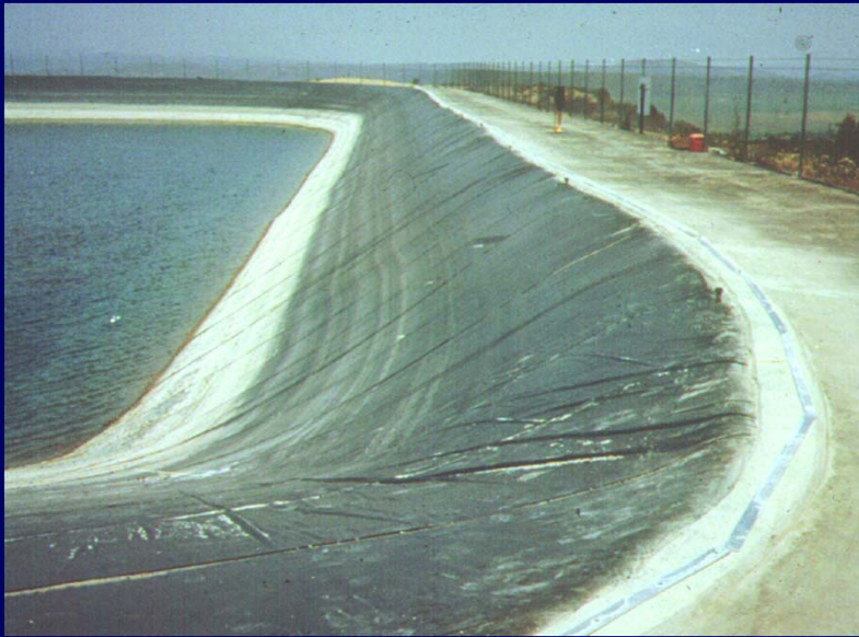
(Lined Potable Water Reservoir)
