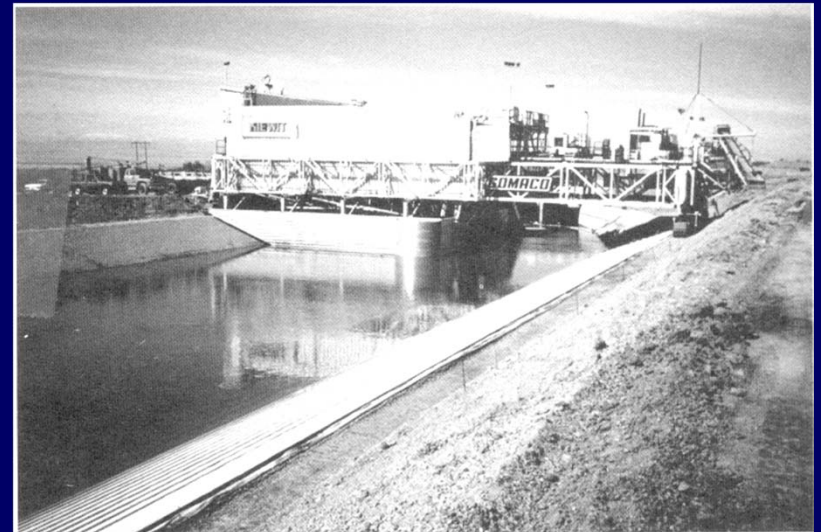
(Lining a "Live" Canal)
