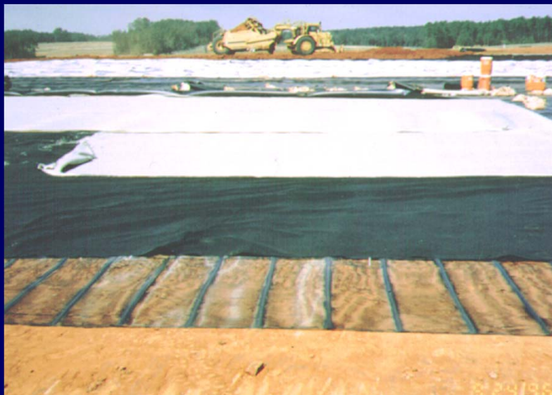
(Seven Layers of Geosynthetics)
