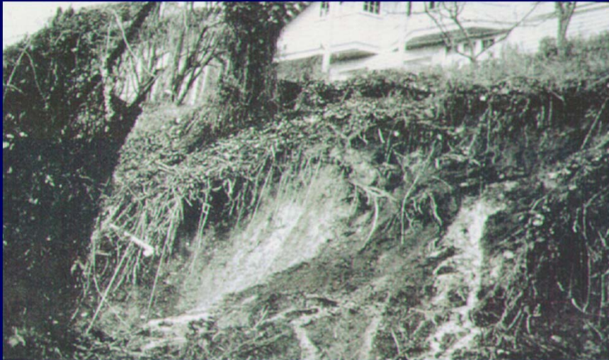
(One that Failed)!
