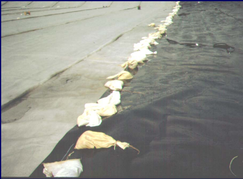
(Secondary Composite Liner)
