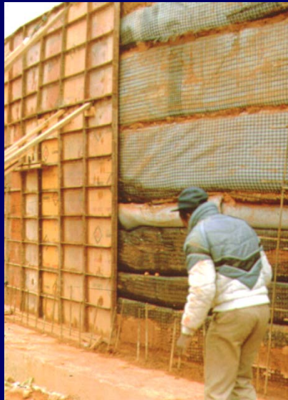
(With Concrete Facing)
