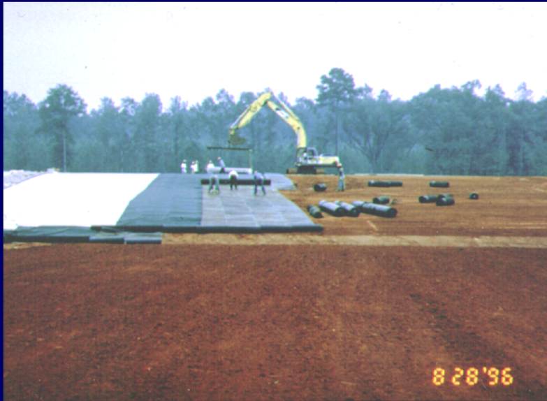
(Sequential Placement of GSs)
