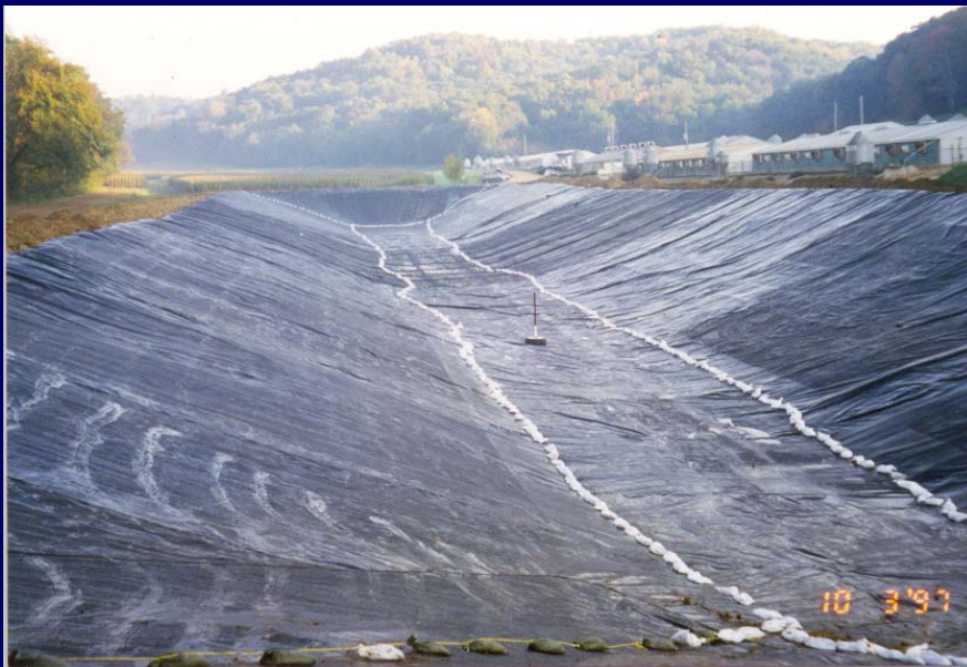
(Lined Pond Behind Cattle Stalls)
