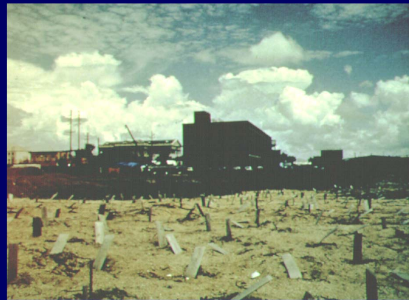
(Ready for Surcharge Fill)
