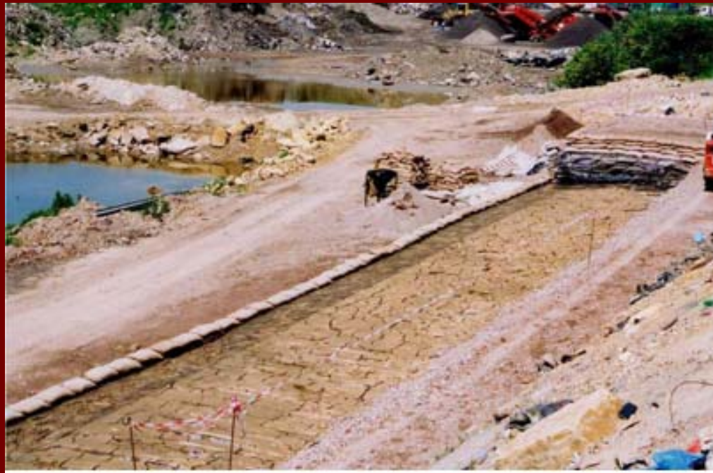
EKG reinforced wall after the construction of lift No. 3
