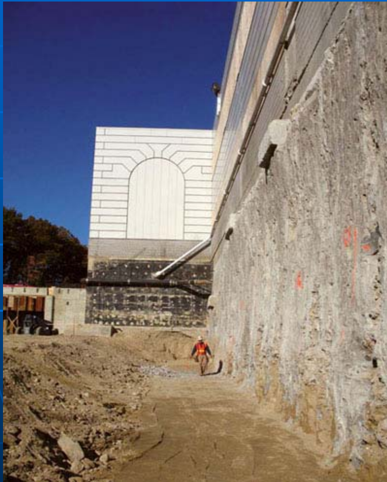
Jet grouted soilcrete columns
