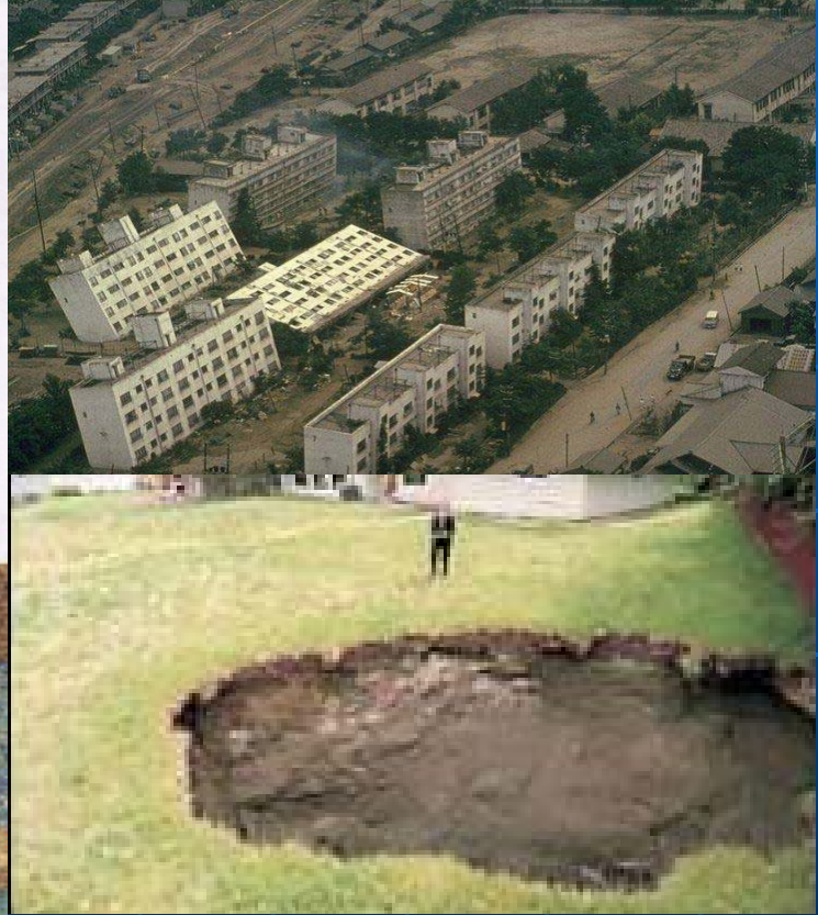
Liquefaction and sinkhole formation
