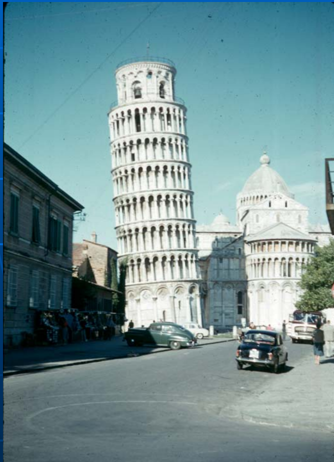
Leaning tower of Pisa
